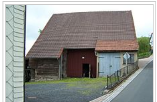
This barn in Thuringia, Germany has two outshots forming the recess to the middle barn doors.
