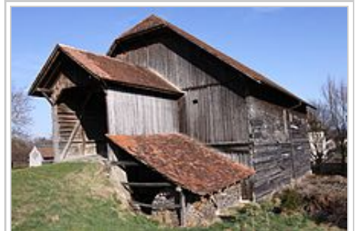
A bridge barn in Switzerland. The bridge (rather than a ramp) in this case also shelters animals.
