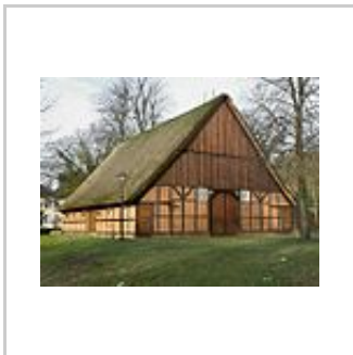
Half-timbered barn with brick infill. Uetersen, Germany. This barn's proportions resemble a Low German house.
