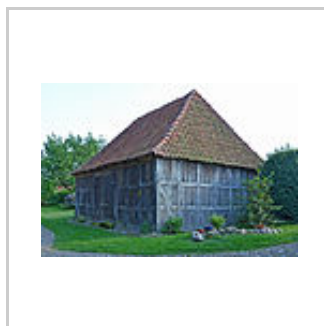
A rare half-timbered barn with board infill in Skye, Lower Saxony, Germany.
