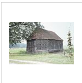
Wattle work walls in a sheep barn in Ruurlo, Netherlands. Image: Cultural Heritage Agency of the Netherlands
