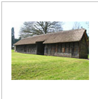
Half-timbered with wattle-work walls for ventilation. Stryd Lydan Barn, originally at Llannerch Banna, Flintshire, North Wales. Re-erected at the St Fagans National History Museum, Cardiff, Wales in 1951.
