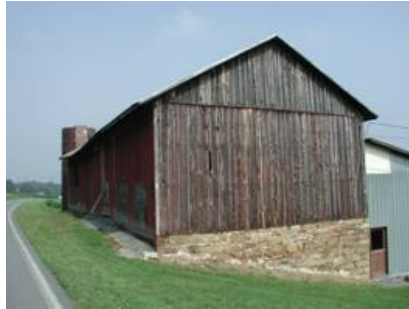
Pennsylvania Barn showing banked construction, Northumberland County, 1845 This barn shows banked construction. Its forebay is enclosed on the gable ends; that is, the foundation extends to the outer edge of the forebay. The barn has a gable roof. This barn has a portion of its original log crib still intact and a date stone of 1845.
