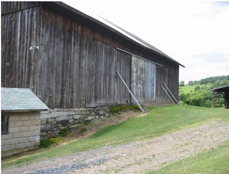
Pennsylvania Barn showing bank side, Columbia County, late nineteenth century This bankside view shows how the ramp led to the central floor. On larger barns, multiple sets of doors led to multiple floors.
