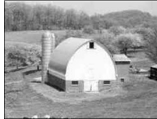
Large Door in Gable End
