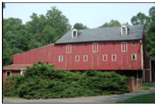
Shed Roof on Gable End
