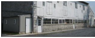
Forebay Enclosed on Eaves Side
