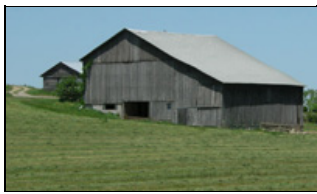
Storm Shed on Stable Level
