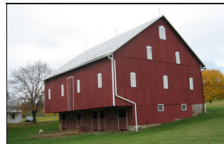
Forebay not Enclosed
