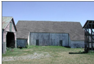
Outshed on Bank Side
