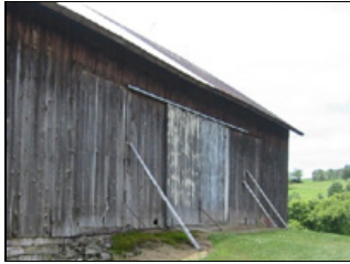
Large Doors in Eaves Side
