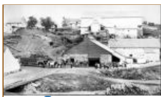
Workers at the Springfield Iron Furnace, Blair County, PA, circa 1870.
