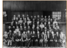
1906 Rolling Mill Crew, Homestead, Pa. United States Steel Corporation. Homestead...
